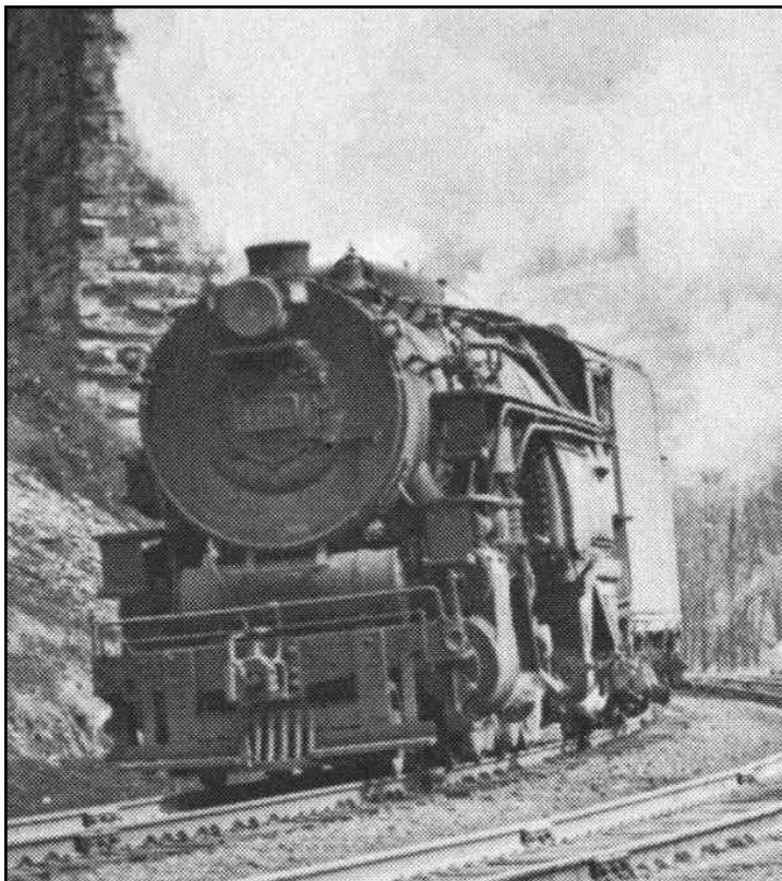
A D&H Consolidation under Starrucca Viaduct
